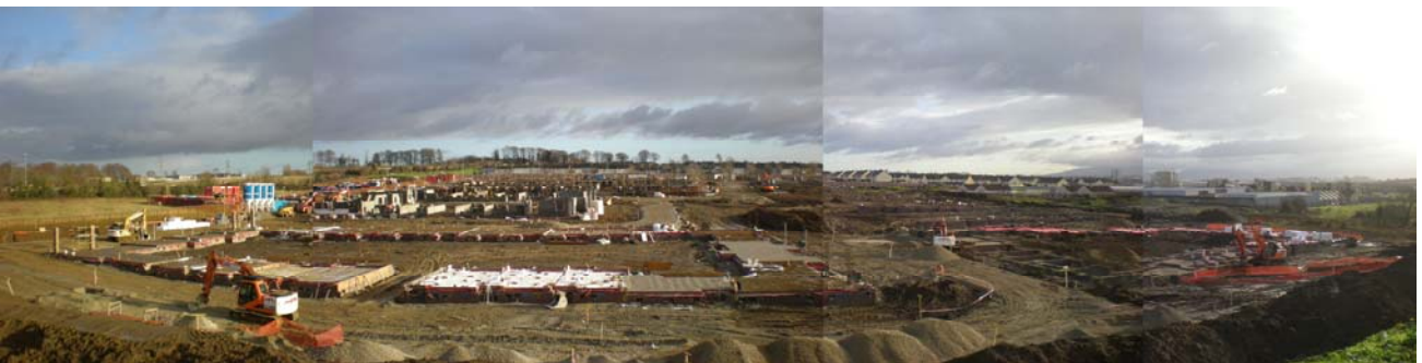
Progress Photographs 09 December 2008
